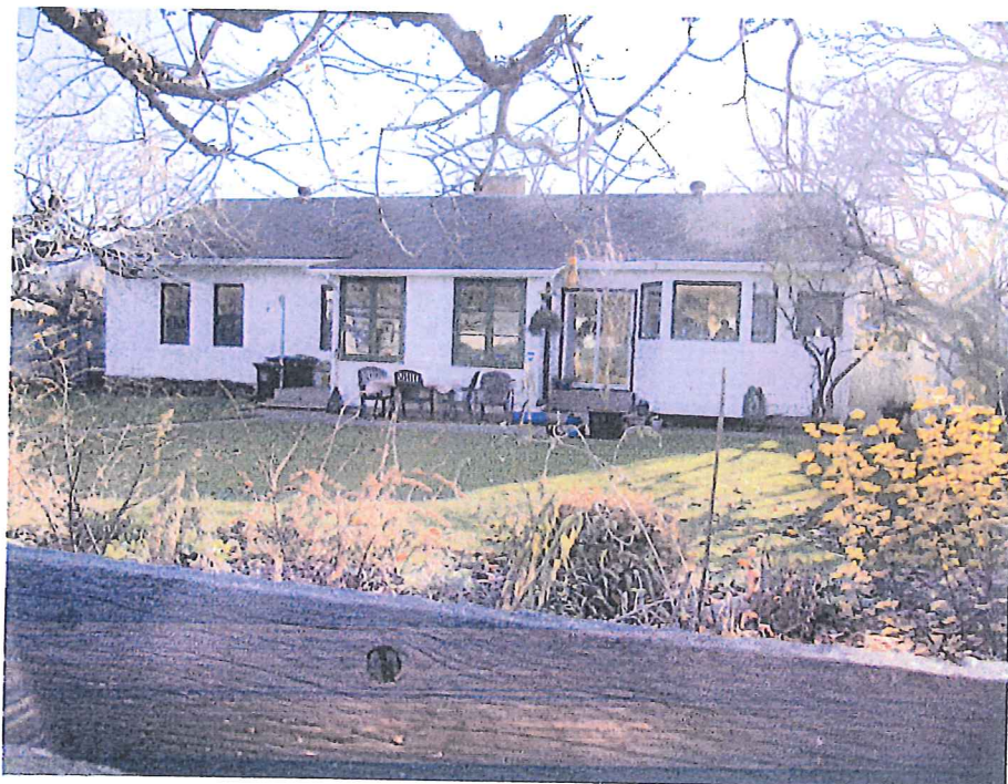
Rear of building. Yard will be paved parking for 10 vehicles. Current vegetation will be transplanted as much as possible to sides of yard along perimeter of paved parking. Rear porch will be removed and replaced with a platform at entrance height (approx 25" from grade). A universally accessible ramp will be built to the East of the platform. Access by steps will be provided to the West of the platform.
